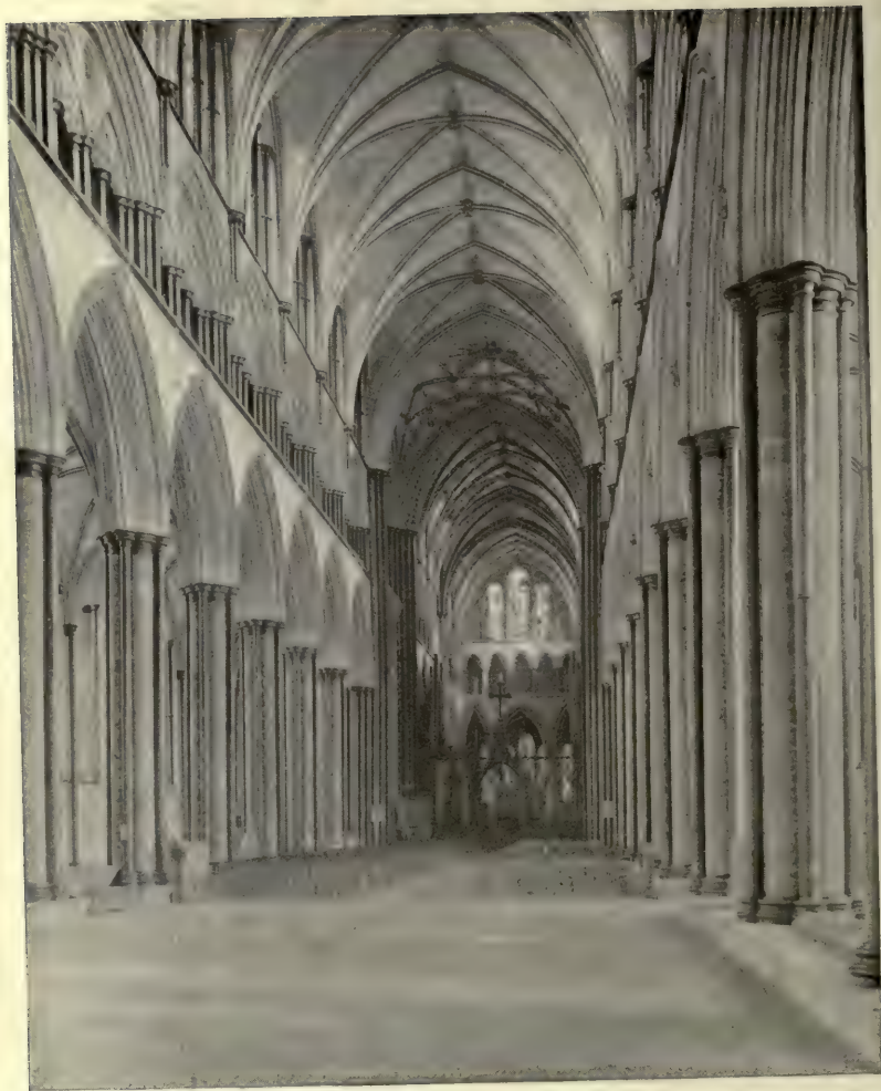
NAVE, LOOKING EAST Cathedral, Salisbury
